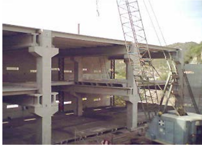
Figure 13: Prefabricated Structure during construction.
